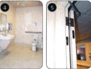
Staff toilet room Staff toilet room door hardware
